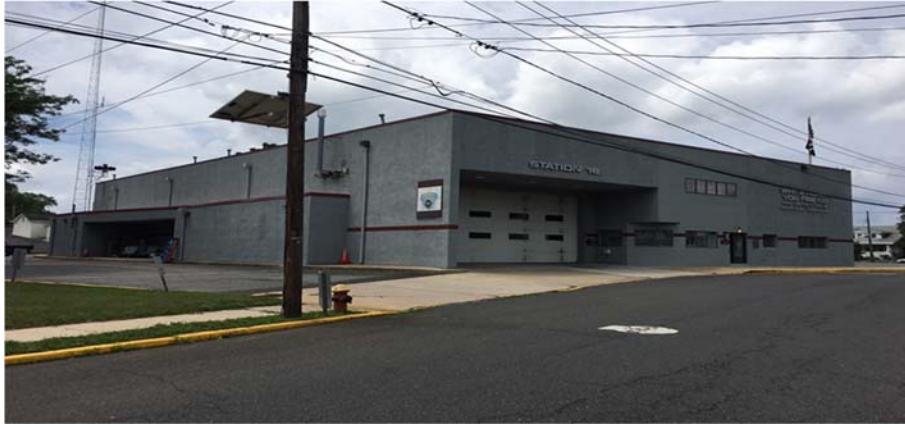
Fire District No. 6, White Horse Fire Company, Station 16, 19 Locust Avenue
