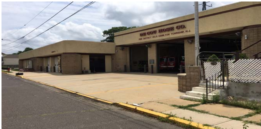
Fire District No. 5, DeCou Hose Company, Station 15, 61 Ruskin Avenue
